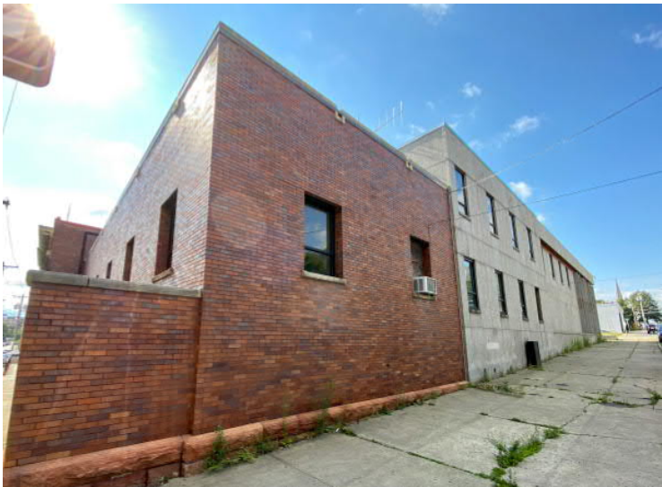
Historic brick exterior and brownstone water table of the South Station building, joining with the granite cladding of the Morton Ave portion of the building.
