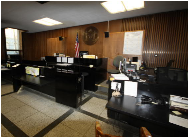
Raised defendant's box does not allow handicap persons to access the box, along with approach clearances.
