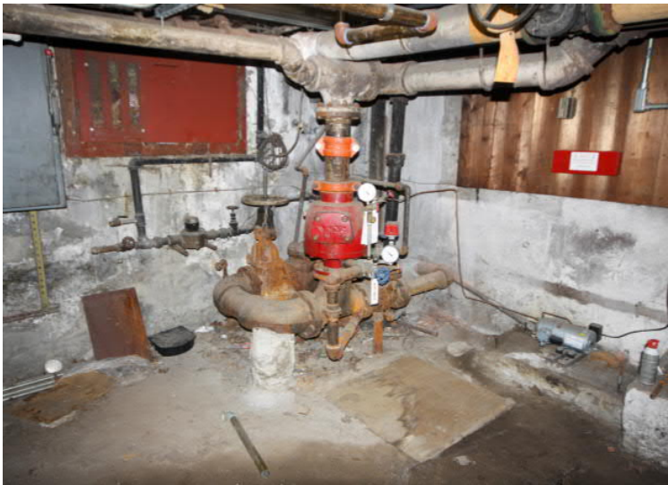
Fire pump in the southeast corner of mechanical room within the South Station portion of the building.
