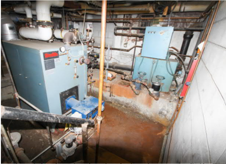
Steam heating boiler within mechanical room located in the South Station section of building.
