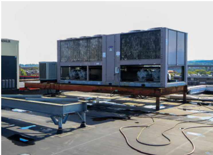
Large central chiller system on the roof that serves the Morton Ave. portion of the building.
