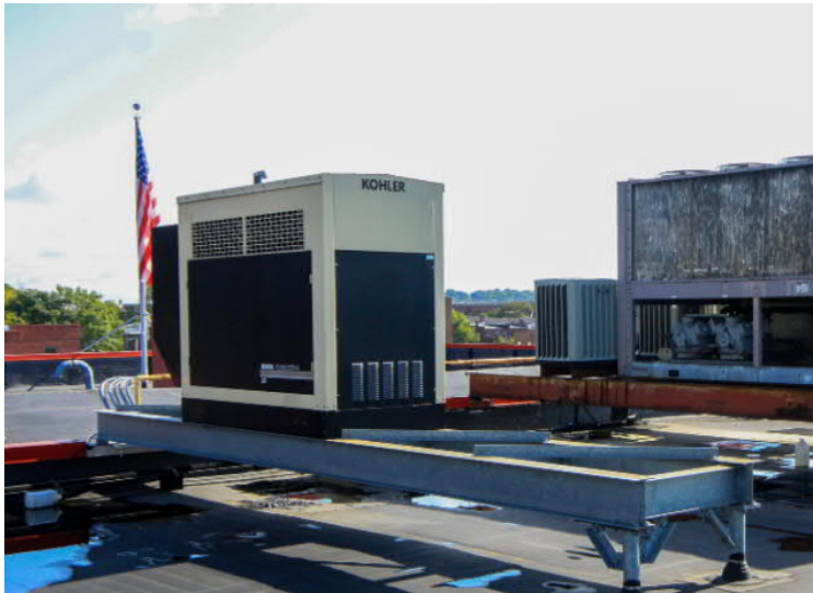
Back-up/Emergency power generator on the roof.
