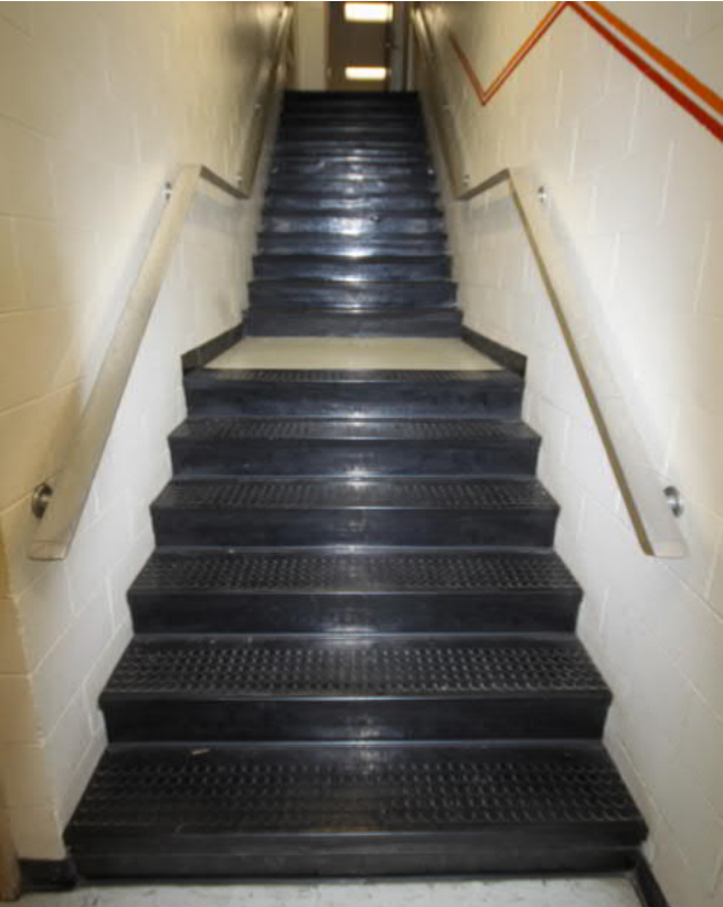
Rubber tread risers and covers installed over stair.
