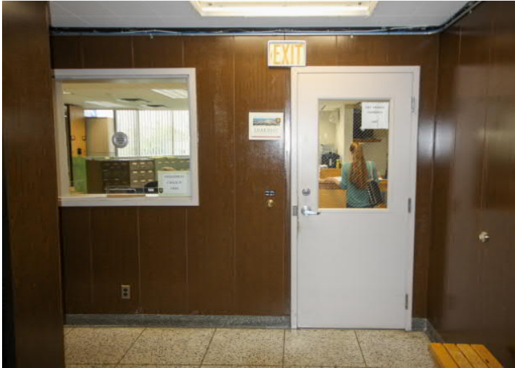
County clerk's existing transaction window does not meet ADA compliance.
