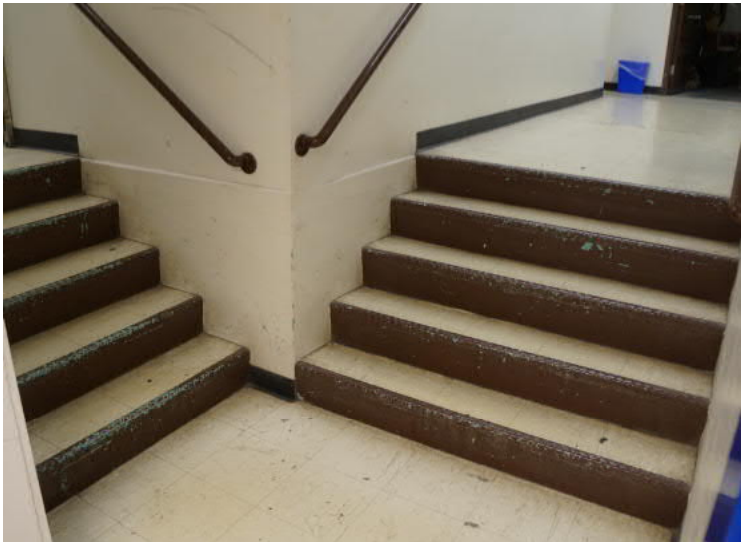
One of many convoluted areas of the building where stairs are installed due to multiple renovations to the interior of the structure creating mid levels.
