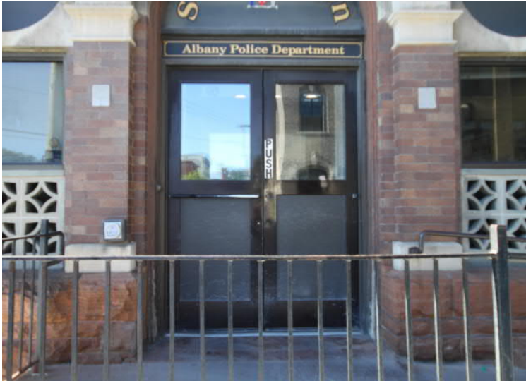
At the entrance of South Station, the double doors swing inward, which to code should swing outward since it is a means of egress.
