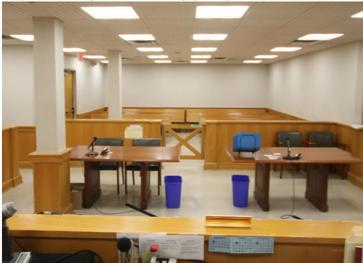
The gate between the benches and seating area is not ADA compliant, making the bench inaccessible to persons in a wheelchair. This does not hold up to the OCA standards of courtrooms.
