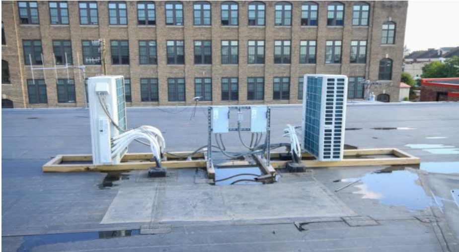
Wood curbing placed directly on top of the roof membrane.
