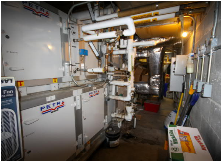
Air handling unit located in a mechanical room on Level 0 that serves some of the adjacent rooms.
