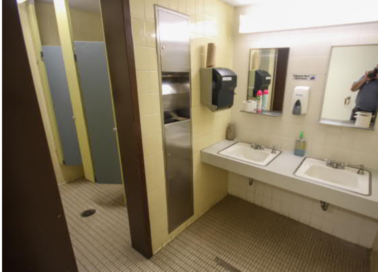
View of the exisint public women's restroom. This bathroom does not meet ADA compliance, failing to have a handicap stall and does not have proper sizing for turnaround clearance.
