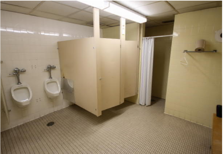
Outdated fixtures and finishes, along with non-ADA compliant urinal, stalls, and shower.
