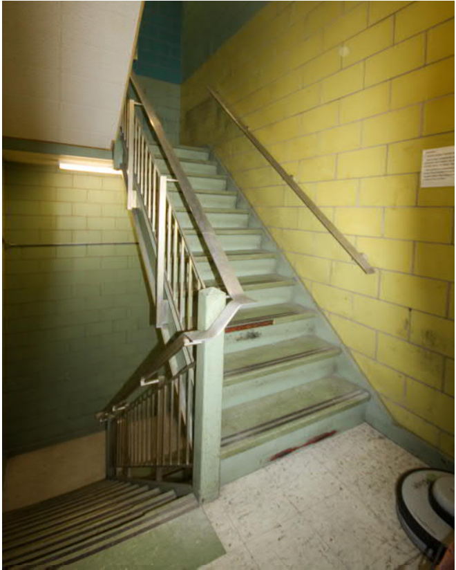
Throughout the building there are many stairways without proper sized areas of refuge for egress stair landings to serve the building's upper floor occupant loads.
