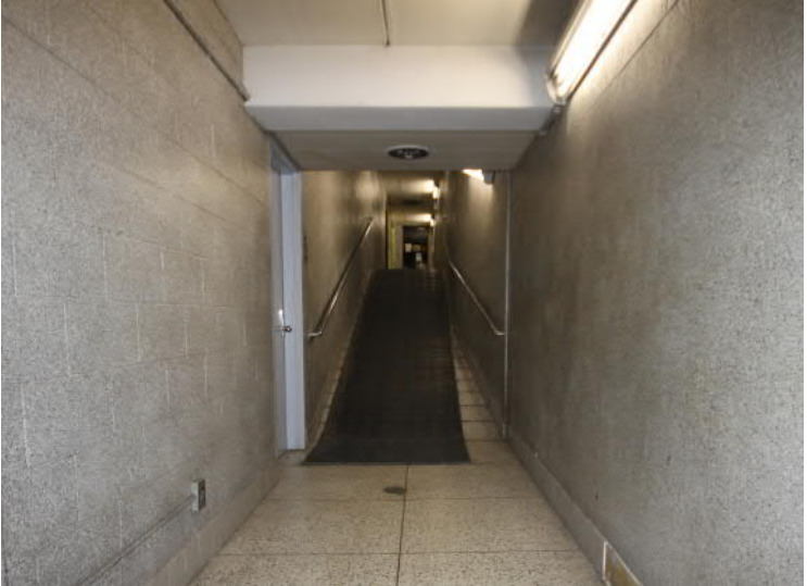
The existing ramp leads from Level 1 to Level 2, bringing incarcerated persons from the holding cells up to the courtrooms. The ramp is not accessible and should contain a landing.
