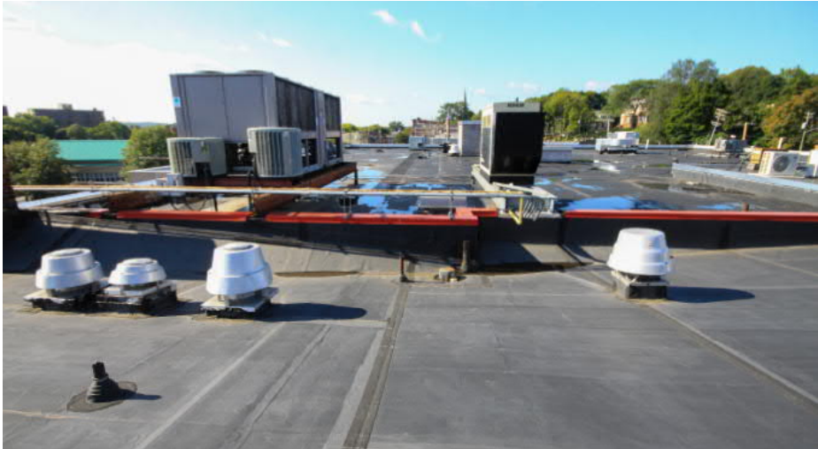
Transition between South Station sloped roof and Morton Ave. EPDM roof.
