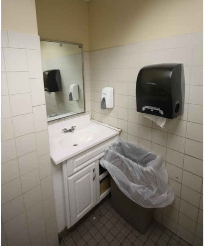
Existing restroom on Level 1, off of the South Station lobby. The sink would not be accessible to a person in a wheelchair, as well as the soap dispenser, and the paper towel dispenser should be mounted high to prevent someone in a wheelchair from hitting their head while approaching the sink.
