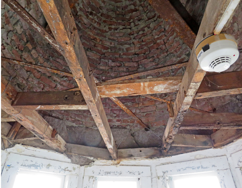
(Above) Tower Stair. Plaster ceiling missing. Steel tie rods rusted and broken. JGWA, 2020.
