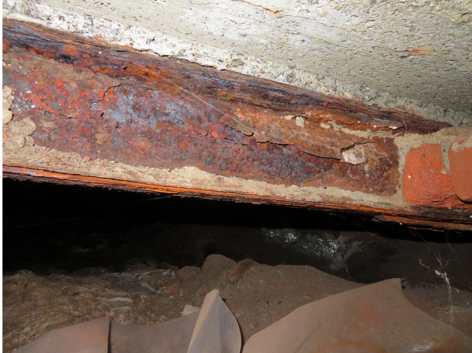
Crawl space below Room 11 (Building Permit Storage). Severely corroded floor beam. The individual brick at the right of the image is from a collapsed brick arch that originally supported the floor. JGWA, 2020.
