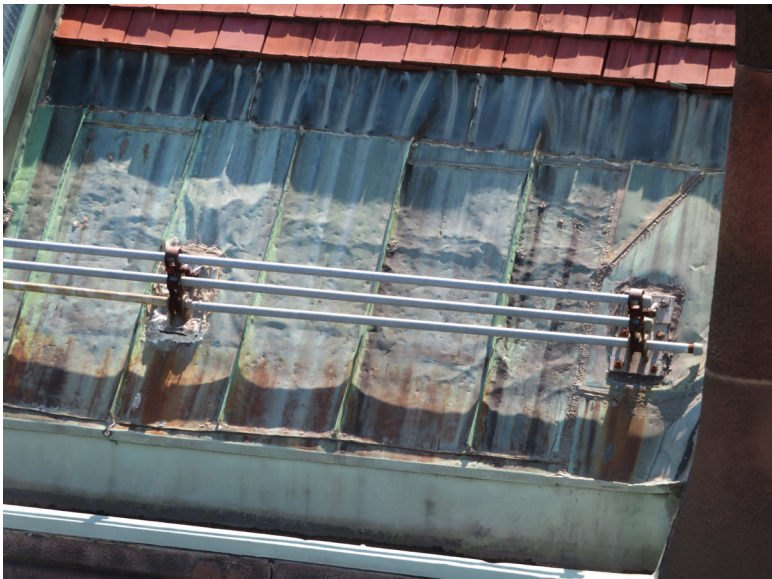
Thin copper deformed by wear and impact damage. Base plates for snow rail provide an access point for water. JGWA, 2019.
