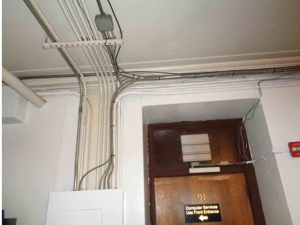
Room 9 (outside Room 91). Wiring secured with cable ties. Unsecured wiring. JGWA, 2020.
