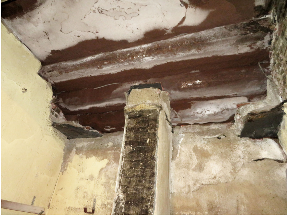
Room 16 (Storage). Deteriorated underside of front entry stairs. Open joints in the stair and foundation have allowed water entry. JGWA, 2019.
