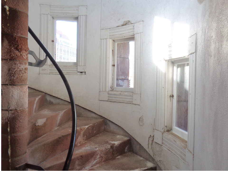
Stair 154C. Plaster damage and evidence of water infiltration on stone stairs. JGWA, 2019.
