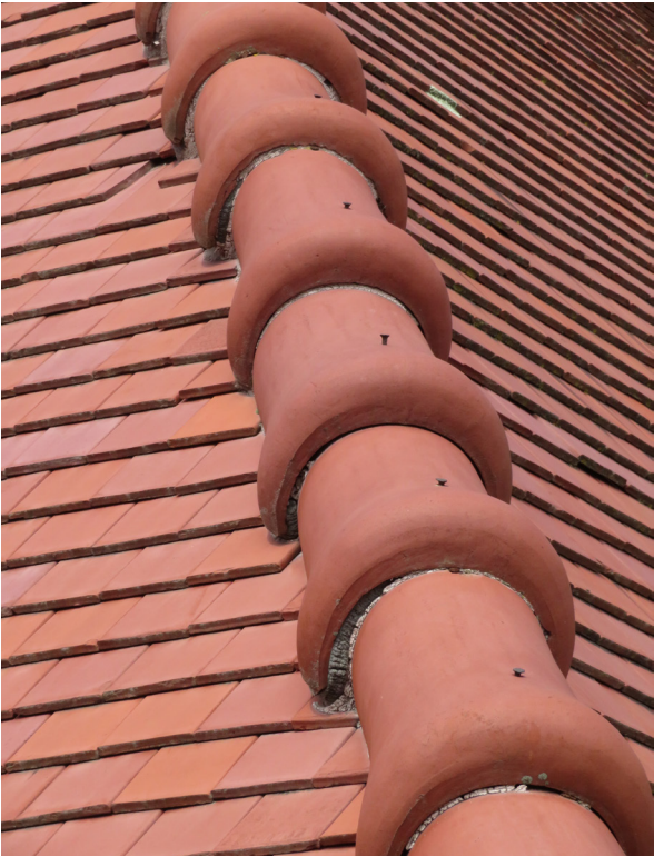
Hip tiles with exposed ferrous metal anchor on northeast hip. JGWA, 2019.
