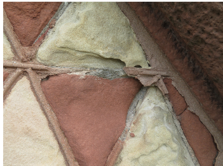
Detail of the stone at the west gable, eroding away from hard 1970s-era mortar. JGWA, 2019.
