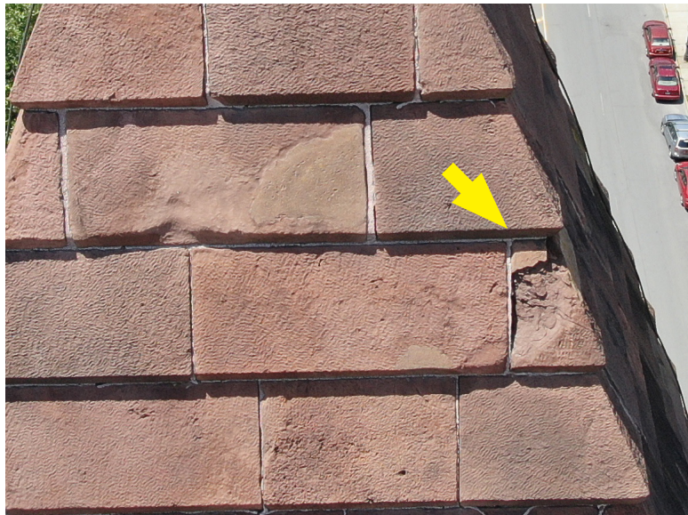
The stone seen above on the east face of the main tower roof has deteriorated badly. A patch from the 1970s work has failed. The surface of the stone to the upper left has eroded substantially. Albany Water Department, 2019.
