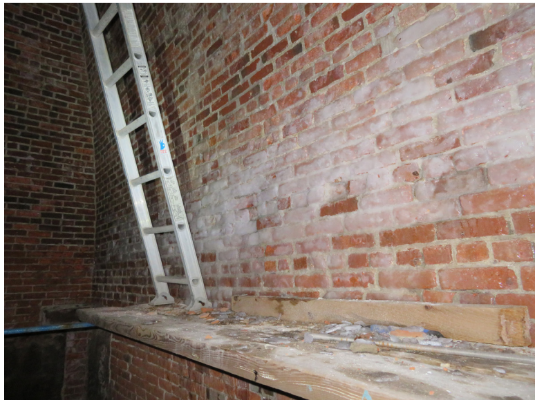
Ice buildup on south face of the interior of tower roof caused by open mortar joints on the exterior. JGWA, 2020.
