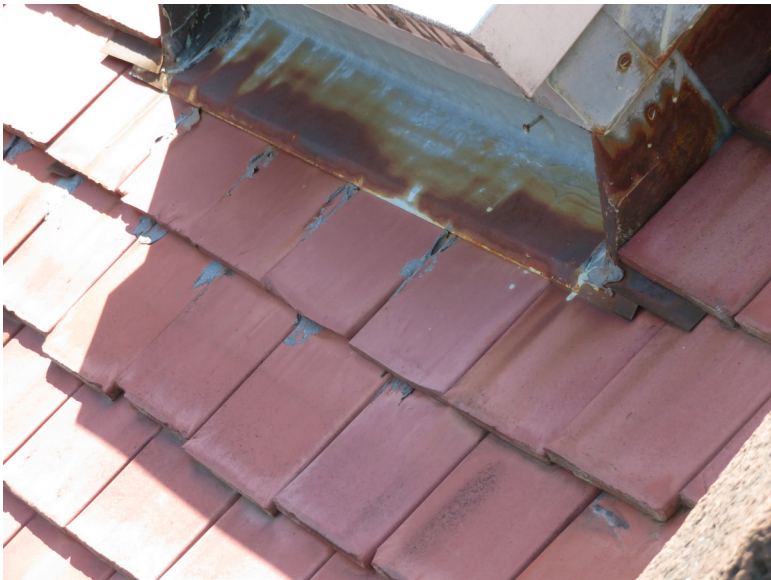
Loose anchors, galvanic corrosion, and loose tiles at base of skylight. JGWA, 2019.
