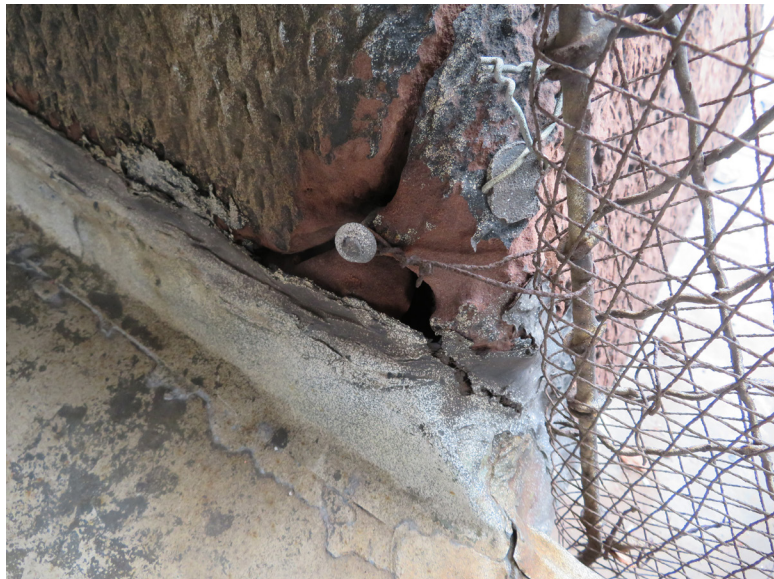
Spalled stone caused by a ferrous metal anchor at the inside of the bell level. JGWA, 2020.
