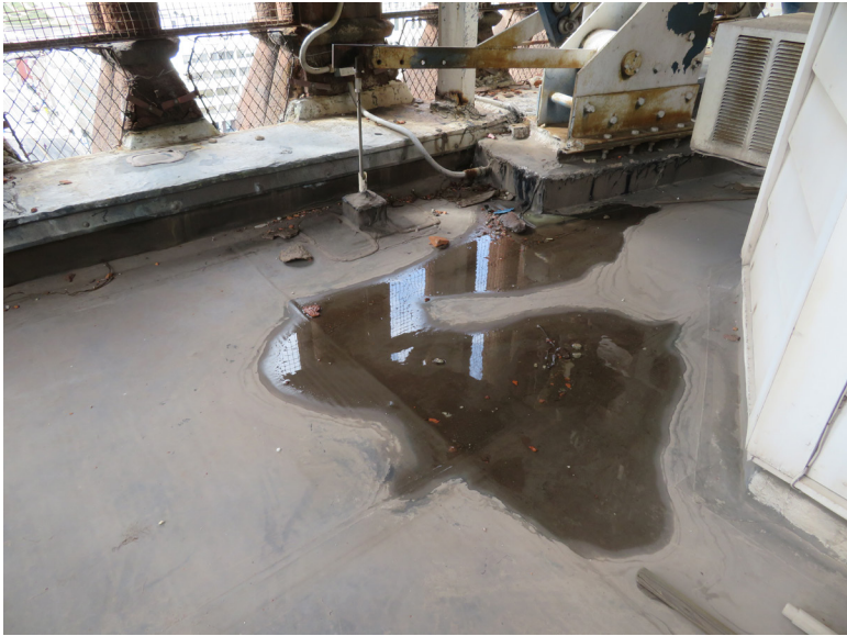
Water collecting at membrane roof at the bell level of the main tower. JGWA, 2020.
