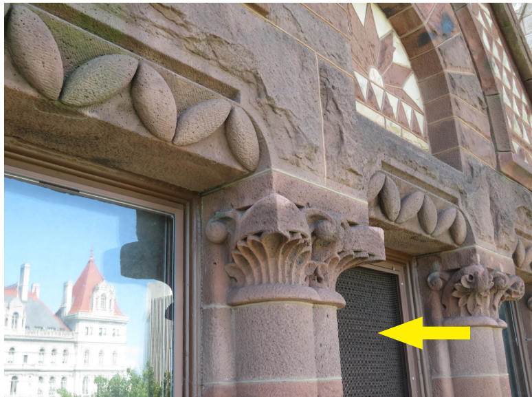
The intake grille at the center of the west gable. JGWA, 2019.
