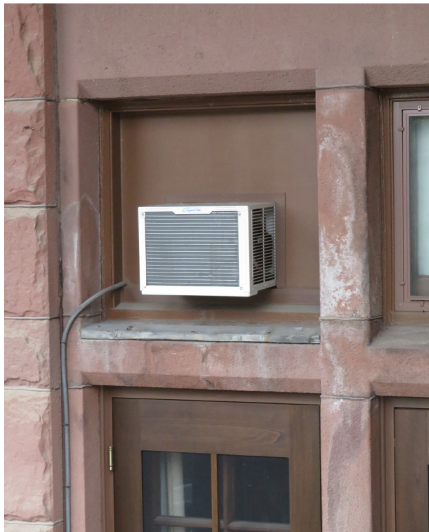
Wood panel and air conditioner over transom window at the loggia. The white haze is efflorescence caused by moisture from the air conditioner. JGWA, 2019.
