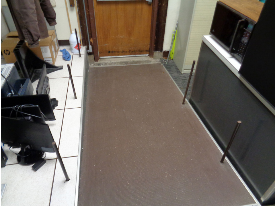
Room 91 (Server Room). Impalement hazard at unfinished or removed railings. JGWA, 2020.
