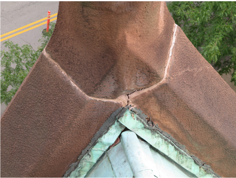
Cap flashings with exposed gap at ridge at north-facing projecting bay. A gap in the sealant and the cracked coping indicate movement. JGWA, 2019.
