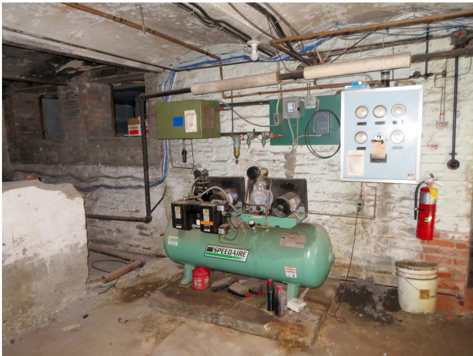
Room 001 (Fan Room). Pneumatic control air compressor. Unsafe electrical connection. Equipment running constantly. Gauges not functioning. JGWA, 2019.
