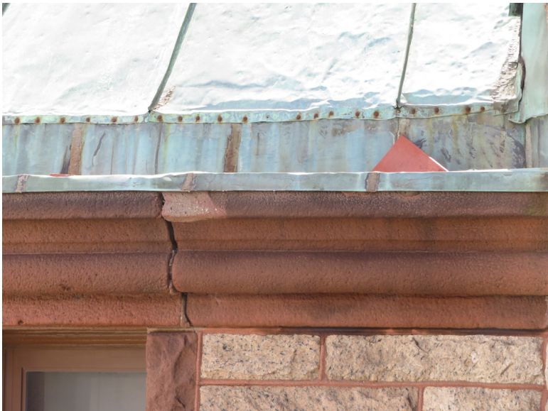
Ferrous nails through face of copper gutter. Roof tile in gutter with patched edge of brownstone below. JGWA, 2019.
