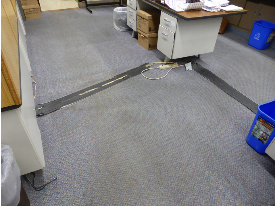
Room 111A (Audit Office). Extension cords taped to worn carpet. Typical in many offices. JGWA, 2020.
