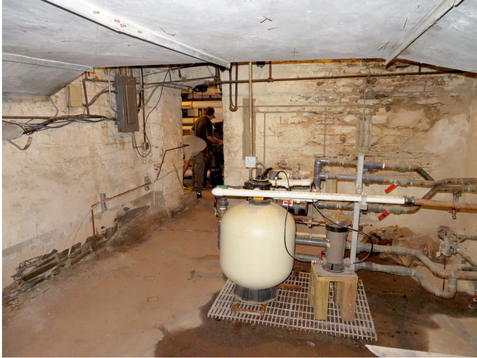
Room 004 (Ash Room). Unsecured wiring and piping. Mortar at masonry walls in fair to poor condition. JGWA, 2019.
