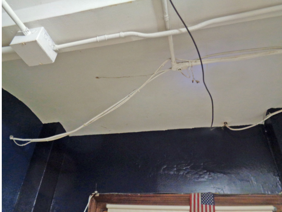
Room 90 (Maintenance). Poorly installed electrical conduit and unsafe exposed electrical wiring. JGWA, 2020.
