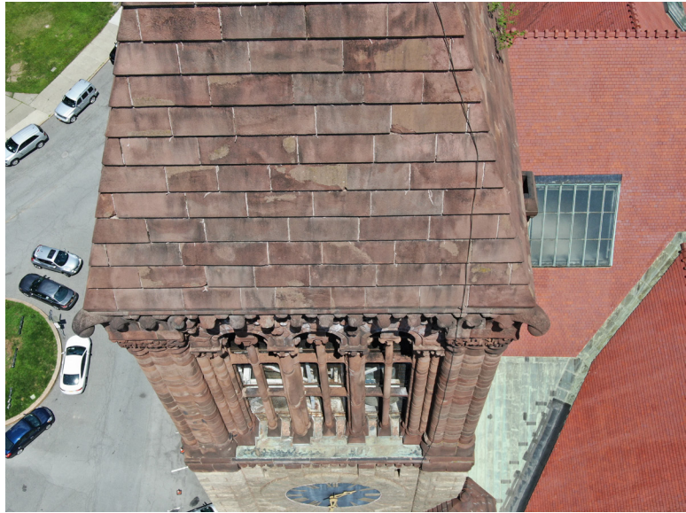
Numerous mortar patches on the south slope of the main tower's brownstone roof. [Image from Albany DGS/Water Dept.]
