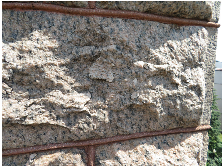
Minor spalling of small areas of the irregular face of the granite. JGWA, 2019.
