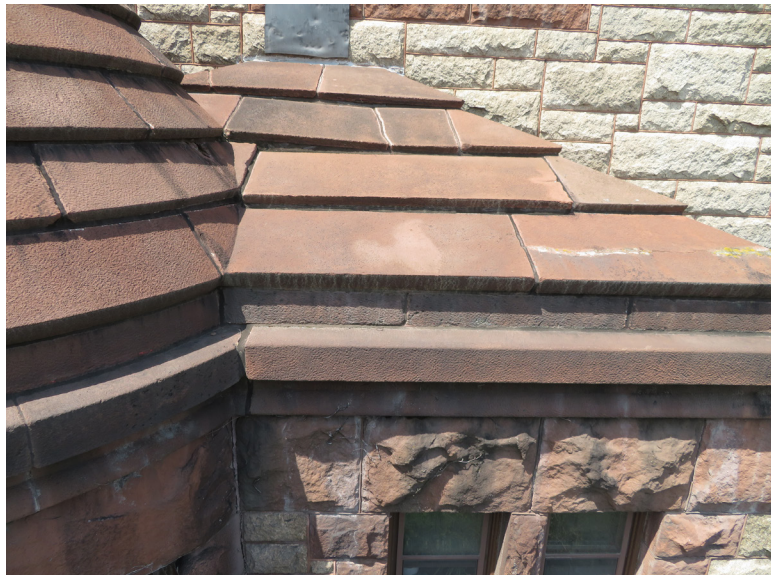
Cracked and displaced stones caused by settlement of the units. The area below was entirely rebuilt in 1916-1920. JGWA, 2019.
