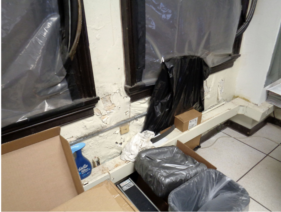
(Above) Room 91 (Server Room). Deteriorated plaster under windows. JGWA, 2020.
