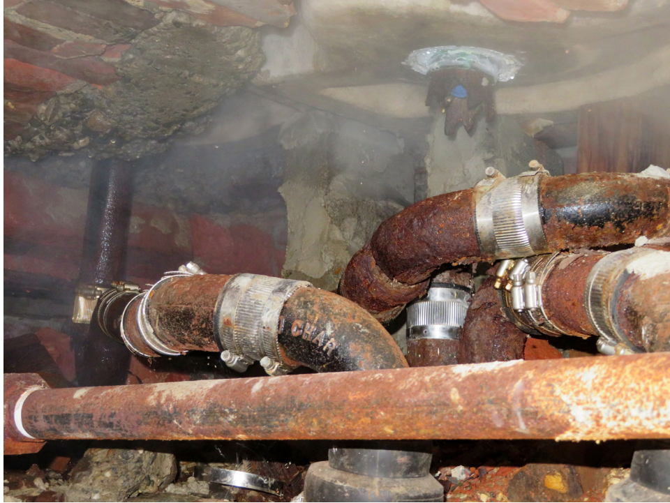
Crawl space below Room 5 (Men's Restroom). Leaking steam heating piping and corroded drain piping. Brick arches have been compromised by holes for piping, and some have partially collapsed. JGWA, 2020.
