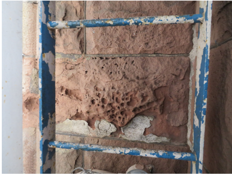
Pitted stone within the bell level of the main tower. The adjacent repairs have not improved the condition. JGWA, 2020.
