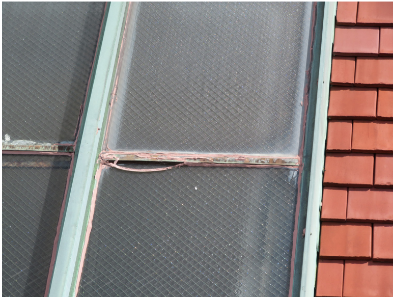
Sealant repairs and sealant failure at south skylight. JGWA, 2019.
