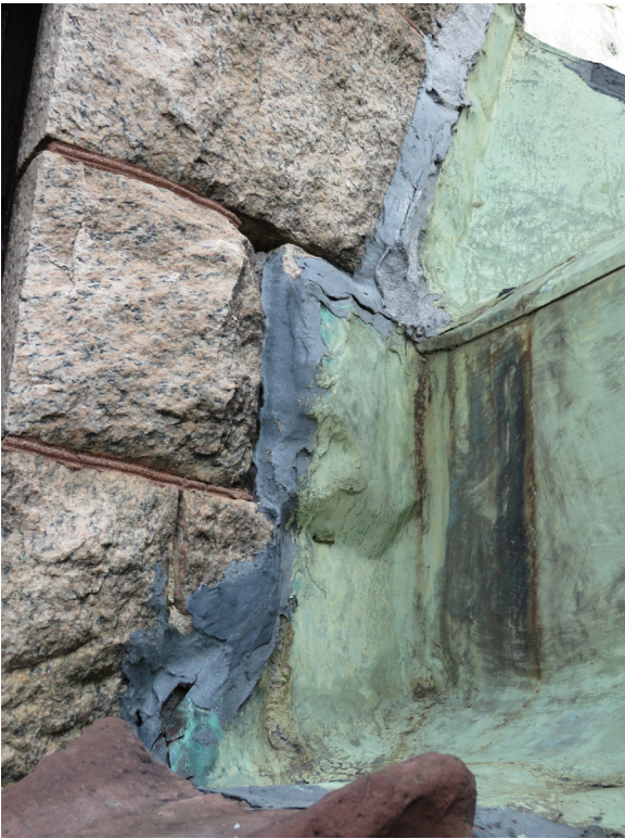
Mastic buildup at the junction of the roof and the east face of main tower and an open mortar joint adjacent. JGWA, 2019.
