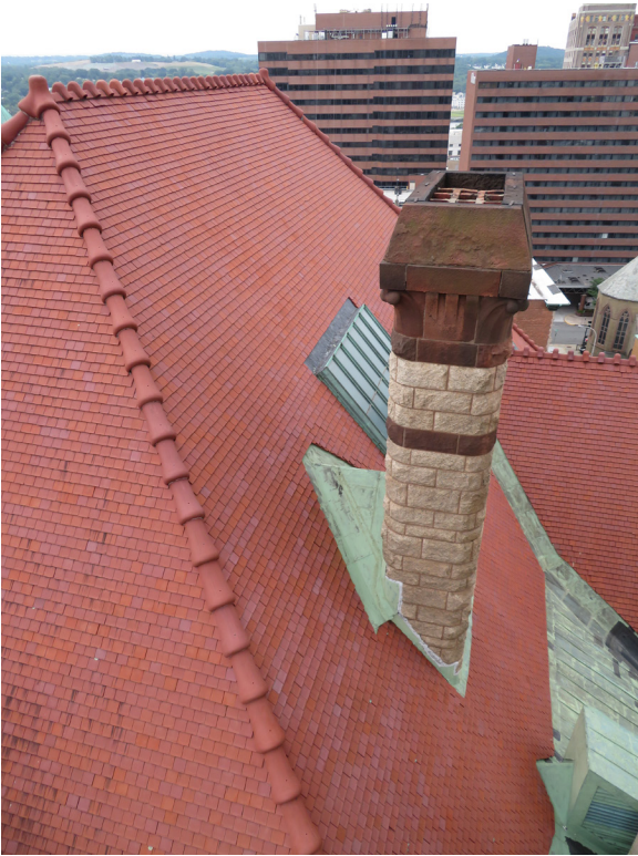
Overview of south slope of roof with chimney, skylight, and large copper-lined valley. JGWA, 2019.
