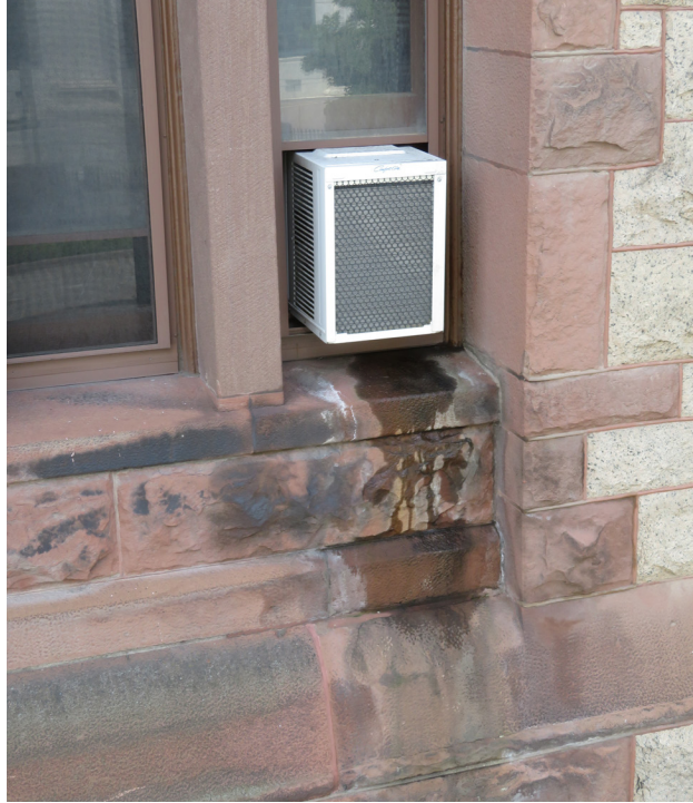
Window air conditioner and condensate runoff with long-term staining adjacent. JGWA, 2019.
