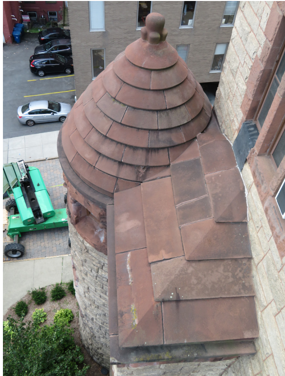
(Left) Cracked and displaced stone in the masonry-built roof on the east-facing projection shows signs of cracks and displacement. JGWA, 2019.
