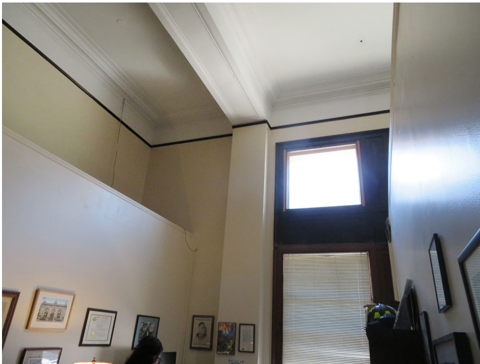
Room 105D (Office). Awkward ceiling configuration caused by the addition of modern partitions in this large historic space. JGWA, 2019.
