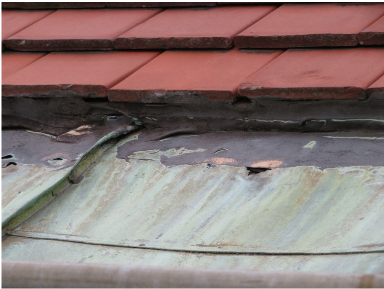
Scoured copper with visible holes where thinned copper has lifted. Mastic has been coated to the bottom of the adjacent tiles in an attempt to stop leaks. JGWA, 2019.
