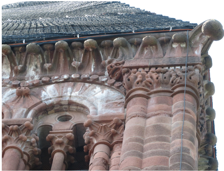
White staining (lime scale) from deteriorated mortar joints at the tower roof and its substructure. JGWA, 2019.
