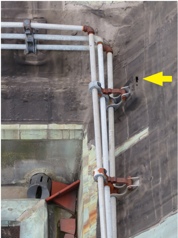
Membrane torn around lifted base plate of displaced snow guard on north elevation. JGWA, 2019.
