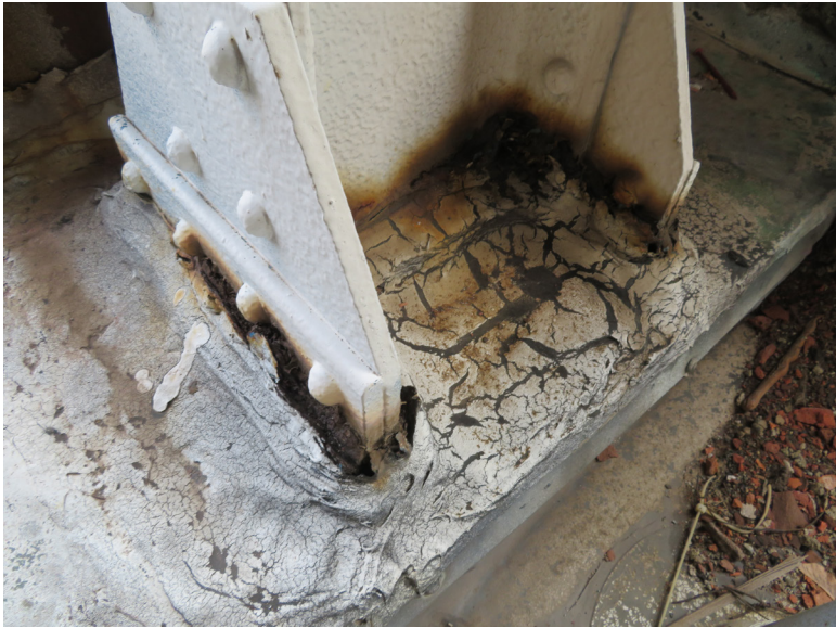
Built up and cracked mastic at base of steel framing bell level of tower. JGWA, 2020.
