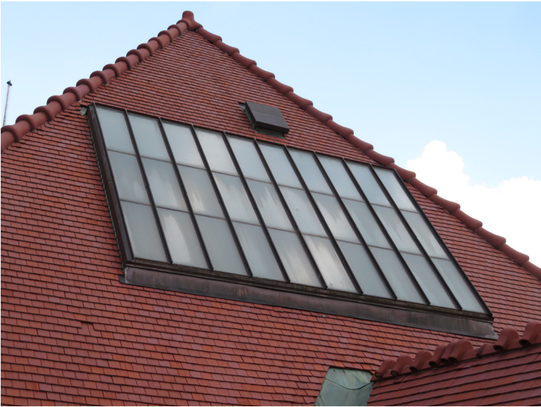
Restored rotunda skylight. The base flashing between the skylight and the roof was not replaced. JGWA, 2019.
