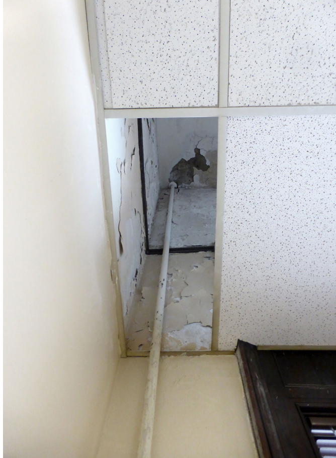
(Left) Room 302 (Assessor's Office). Lay- in ceiling tile conceals water damage above. JGWA, 2020.
