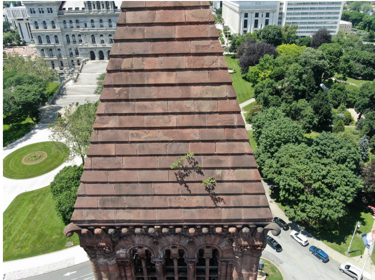
Open mortar joints allow for wood plant growth on the roof of the east face of the main tower roof. These root systems can displace the stone cladding. Albany Water Department, 2019.
