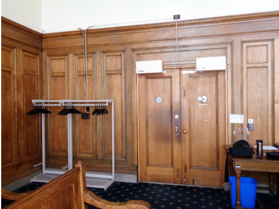
Room 210 (Courtroom). Worn finish and disused tape on doors. Surface-mounted wiring and equipment should be designed to minimize visual impact. JGWA, 2019.
