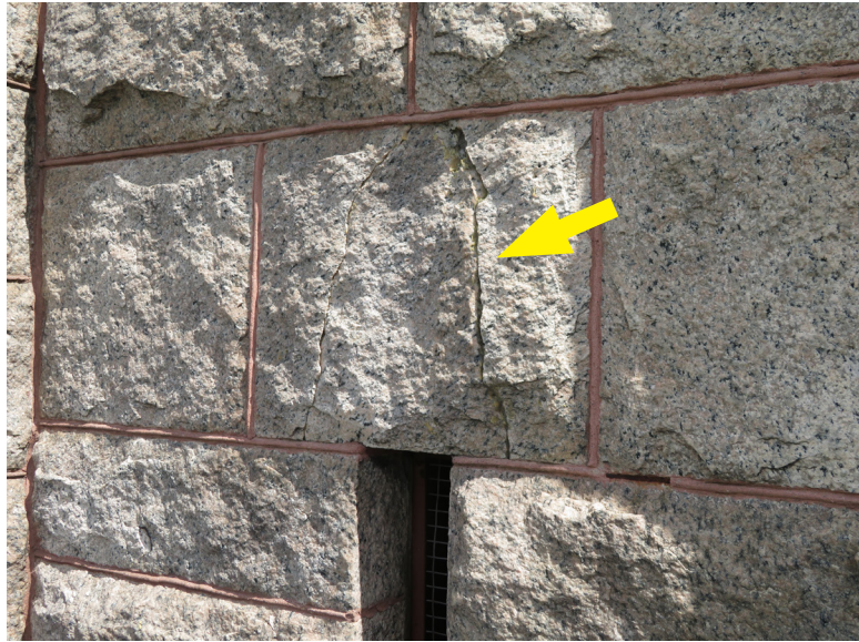
Two cracks, and epoxy repairs, at a granite lintel of a south-facing tower window. JGWA, 2019.
