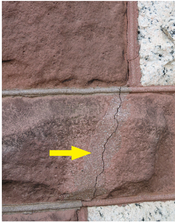
A new crack through an area of repaired brownstone from the 1970s. JGWA, 2019.
