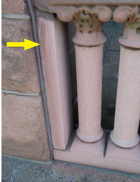
Deterioration along the bedding plane of new stone at loggia balustrade. JGWA, 2019.
