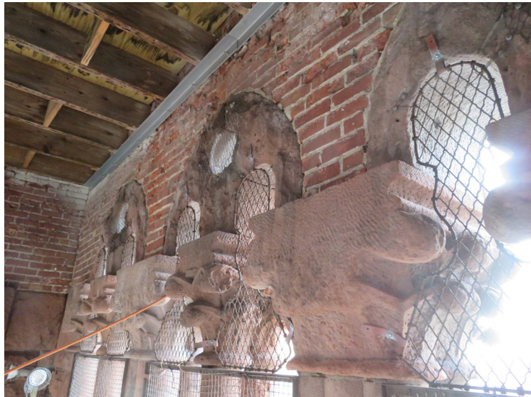
Deteriorated stone in the arches at the top of the main tower. The metal grates are secured with ferrous metal anchors that have caused spalling of the stonework in some locations. JGWA, 2019.
