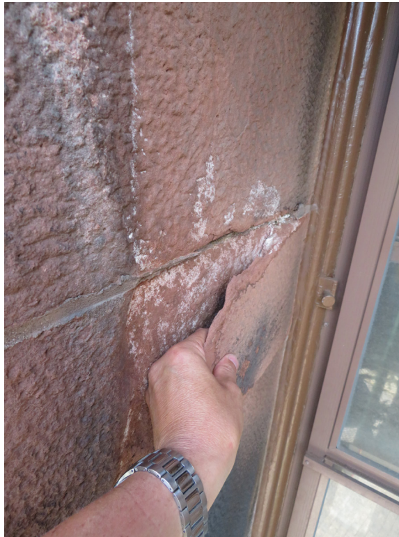
Spalled stone at south-facing window jamb. The loose piece was removed for safety. JGWA, 2019.
