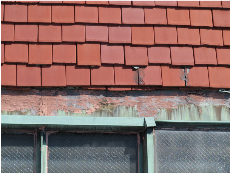
Mastic and missing cap flashing at head of south-facing skylight. Several terra cotta tiles have dropped out of position. JGWA, 2019.
