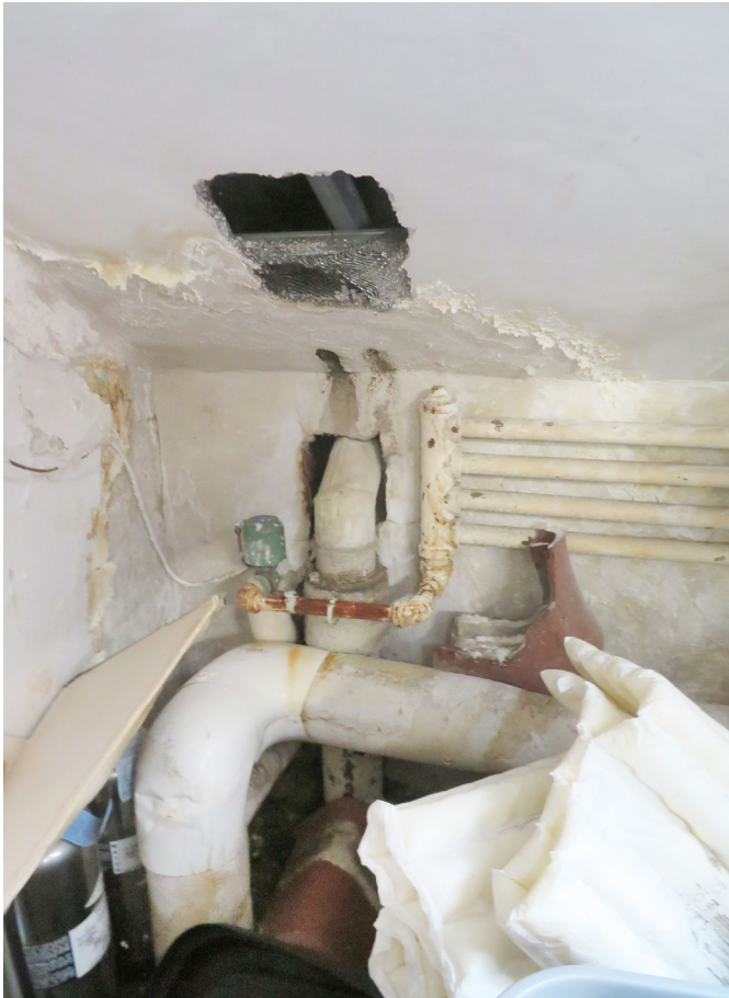
(Above) Room 205E (Office). Water staining and damage from leaking masonry-built roof. JGWA, 2020.
