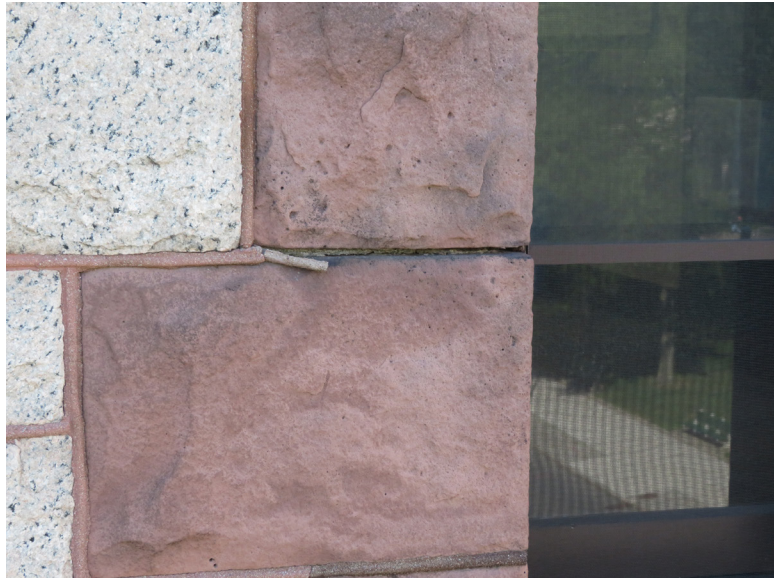
Mortar failure at mildly deteriorated brownstone. JGWA, 2019.
