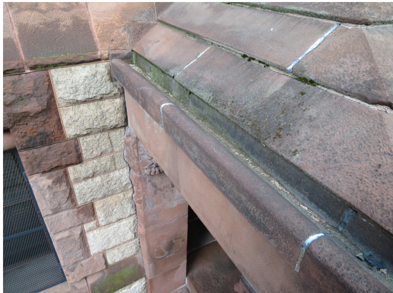
Moss buildup in joints and debris in stone gutter at south entry porch. JGWA, 2019.
