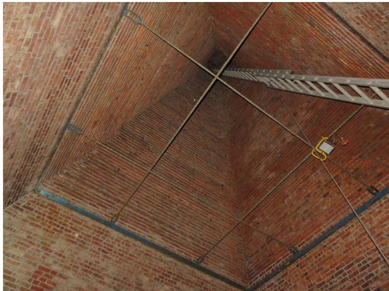
The corbeled brick interior of the main tower roof. JGWA, 2020.
