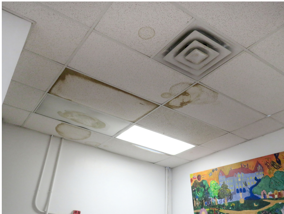
(Below) Room 407 (Lobby). Water damage from leaking skylight above. The historic skylight is completely obscured from view. JGWA, 2020.
