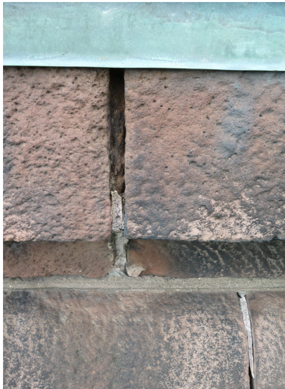
Sealant and mortar failure adjacent to a gutter. JGWA, 2019.
