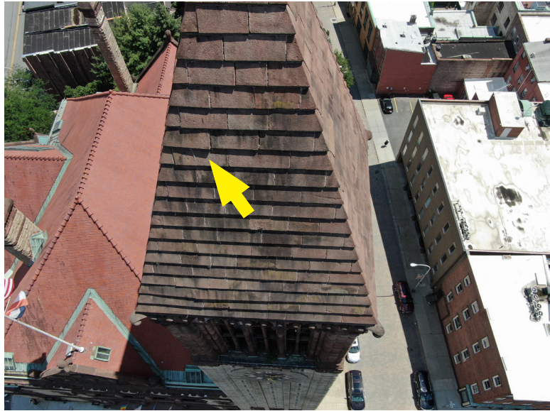
Displaced cladding stones in the west face of the masonry roof of the main tower. Most joints in this roof have failed and provide multiple routes for water ingress. [Image from Albany DGS/Water Dept.]
