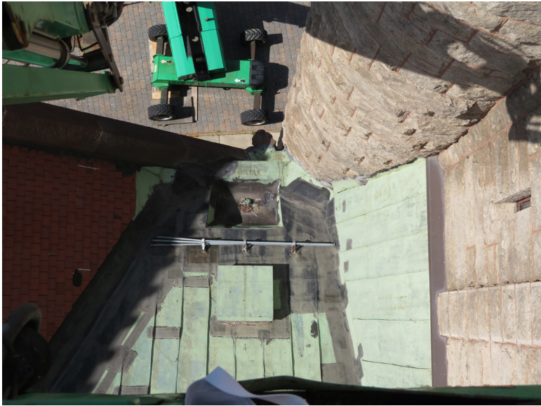
The complex and troubled valley between the main tower and the south gable. JGWA, 2019.
