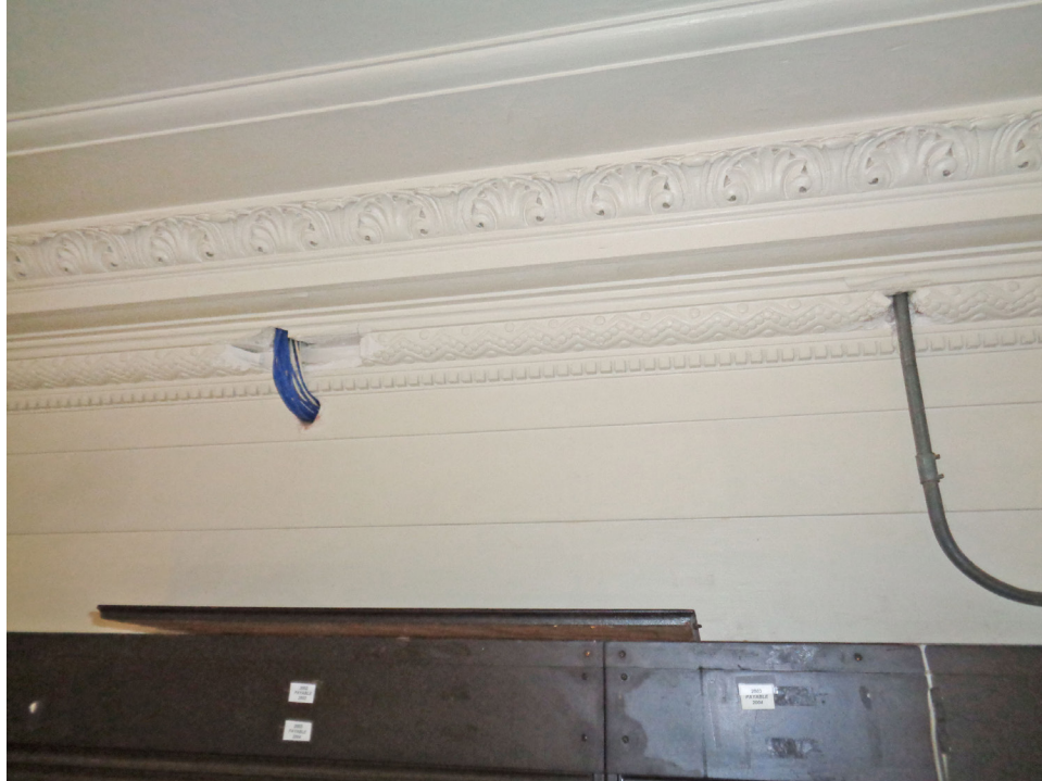
Room 150 (City Treasurer Mezzanine). Decorative plaster cornice damaged by wiring installation. This space is highly visible from publically-accessible Room 110. JGWA, 2020.
