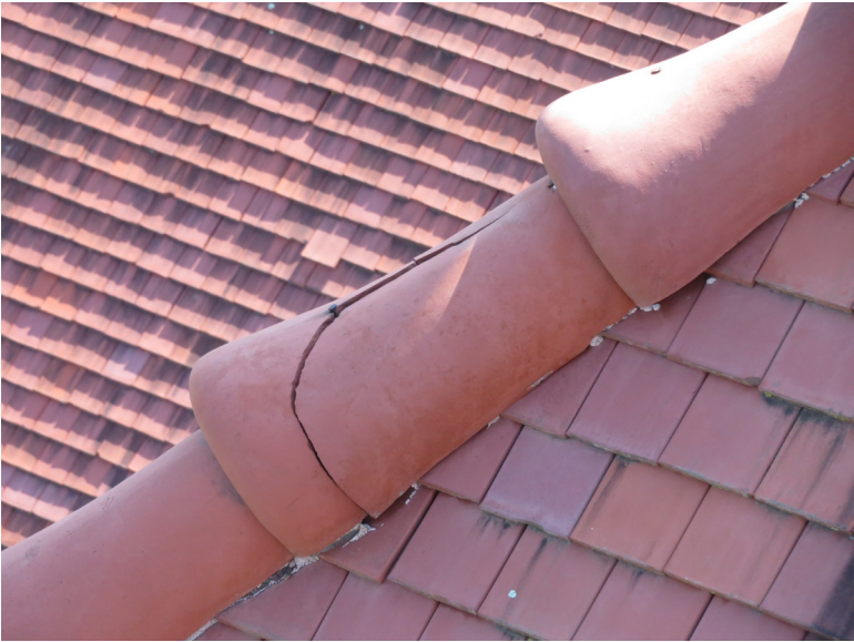
Badly cracked hip tile at northwest hip. JGWA, 2019.
