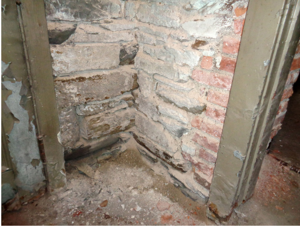
Room 003 (Vestibule). Mortar washed out of joints. JGWA, 2020.
