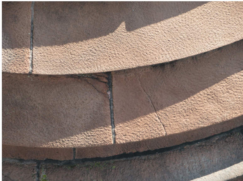
Cracked roof stones and failed joints at southeast tower. JGWA, 2019.
