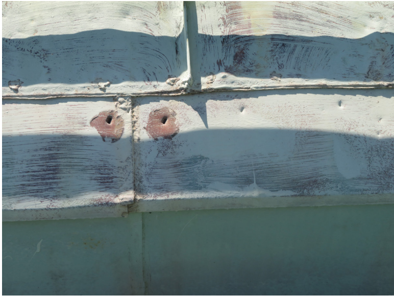
Holes in copper above gutter. JGWA, 2019.
