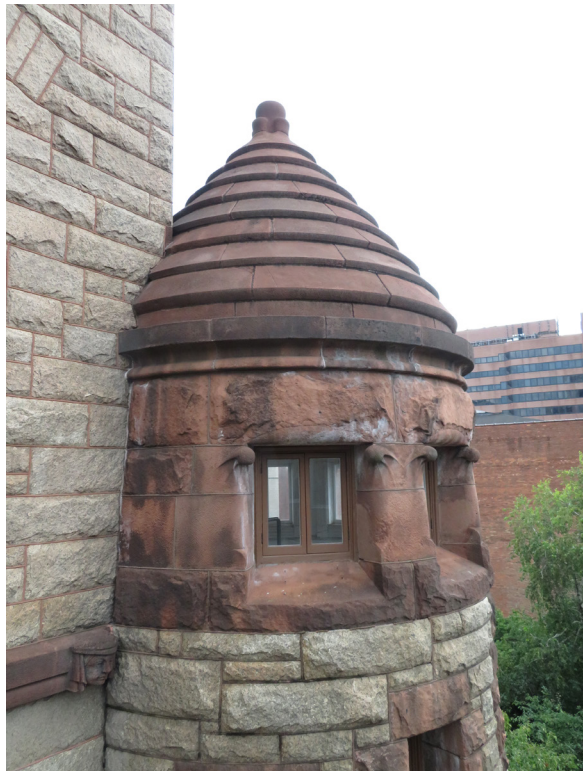
The southeast tower roof with signs of water runoff below the cornice where there is no drip edge. JGWA, 2019.
