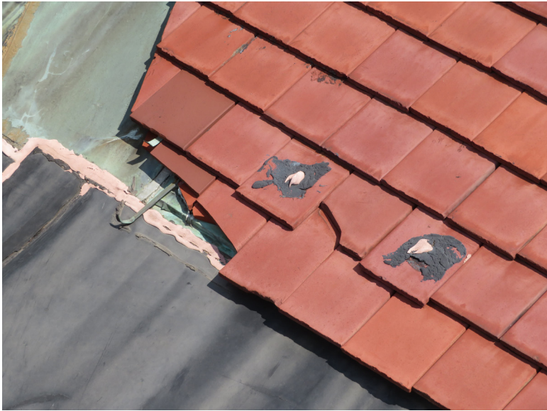
Broken and patched terra cotta roof tiles and membrane patch on top of worn copper roofing. JGWA, 2019.
