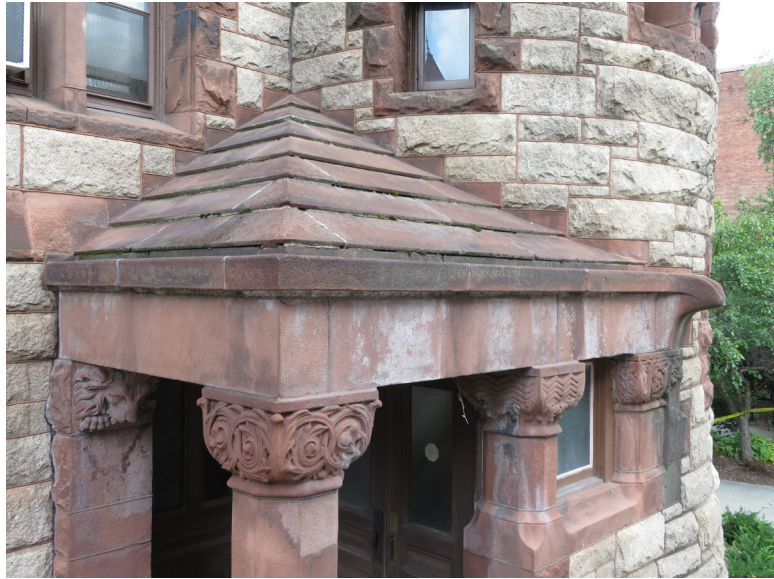
South entry porch roof. Joints have been filled with lead wool in 2006. JGWA, 2019.
