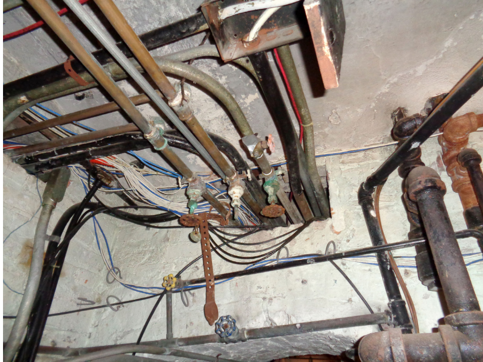
Room 004 (Ash Room). Unsecured piping and wiring. Open junction boxes. Corroded valves. JGWA, 2020.
