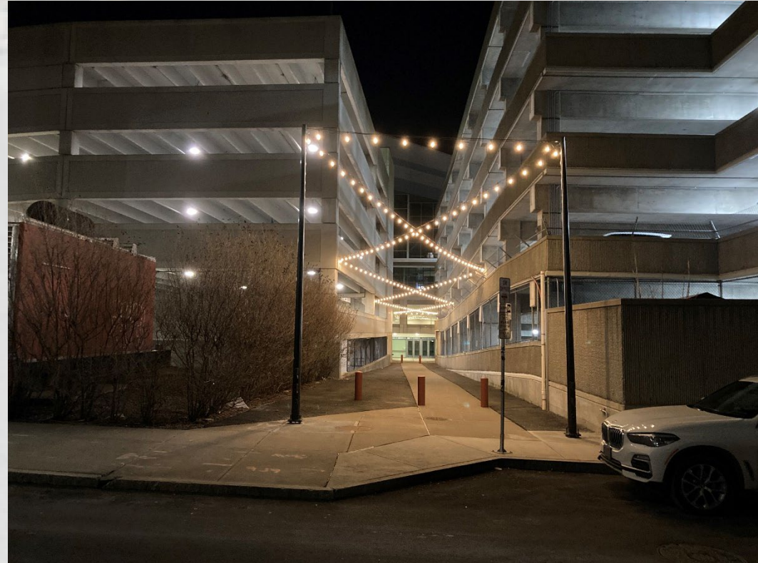
Recent Light Installation on Williams St.
