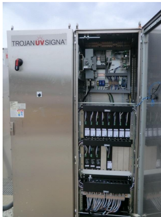
Figure 2-3 Ballast Cabinet (Trojan Technologies TrojanUVSigna™)
