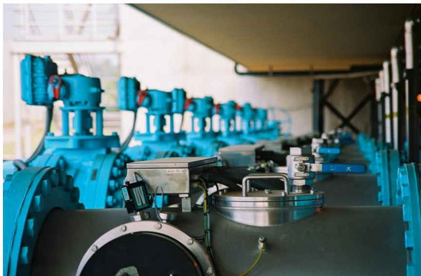
Figure 2-7 Closed-Vessel UV System at R.L. Sutton WRF, Smyrna, Georgia
