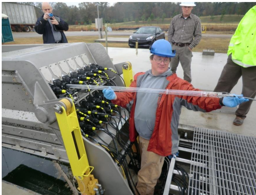
Figure 2-6 Inclined, Open-Channel UV System at H. C. Morgan WPCF, Auburn, Alabama (UV module raised to service position)
