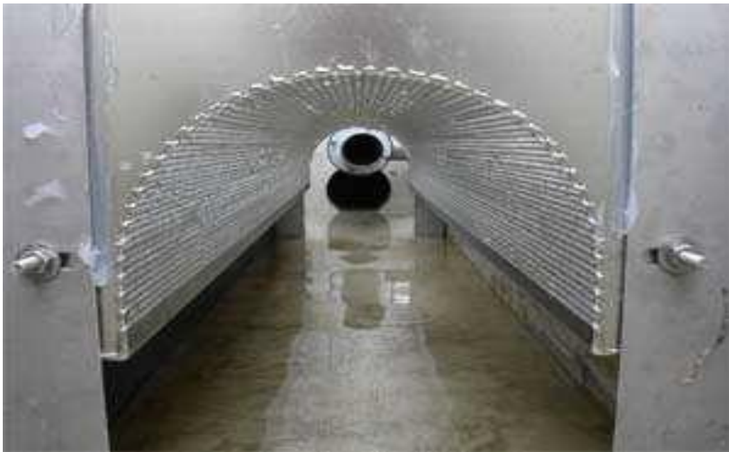
Figure 2-15: Pump Action Screen (CSO Technik)
