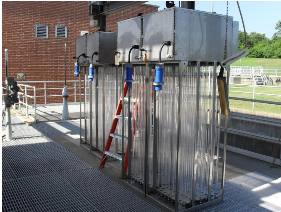
Figure 2-5 Vertical Open-Channel UV System at Massard WPCF, Fort Smith, Arkansas
