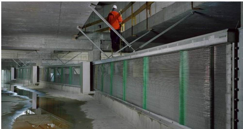
Figure 2-9: Mechanically Raked CSO Bar Screen (Westech ROMAG) – Vertical Screen Installation
